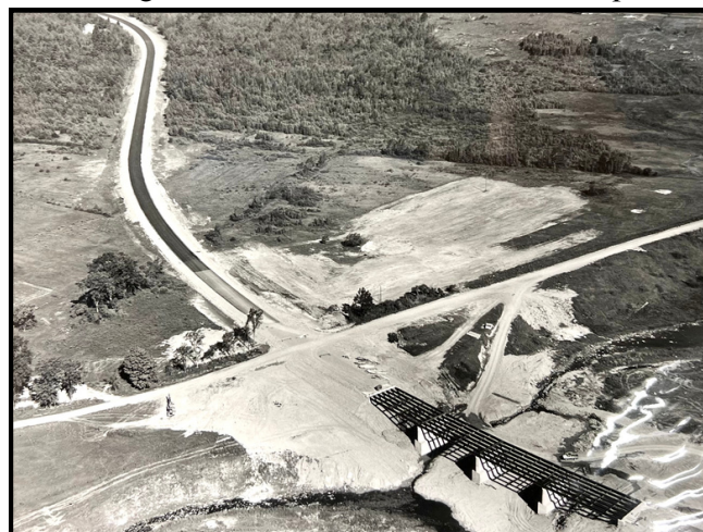
Building the bridge across Brandy Brook on the relocated Route 37.
