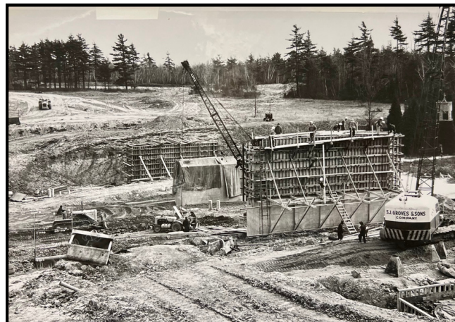
Rerouting Route 37; two more photos showing the construction of the new bridge over Brandy Brook.
