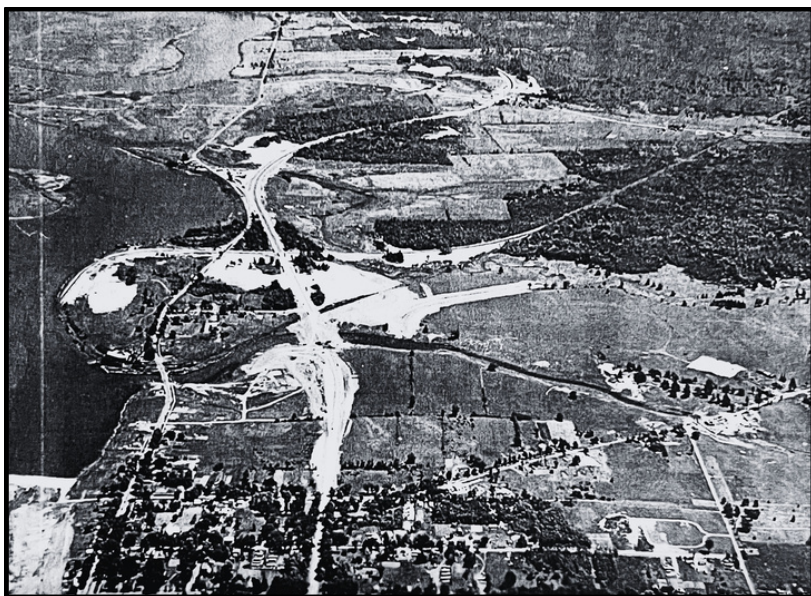
Relocating Route 37 - Aerial view of the new road going through Waddington toward Massena over a new bridge on Big Sucker Brook. The photo gives you an idea of how much land had to be taken along the river after the new road was opened.
