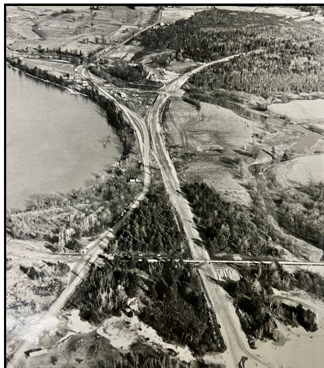
The New Route 37 ran parallel to Old Route 37. The St. Lawrence-Norwood railroad line is shown intersecting the roads in the lower half of the photo.
